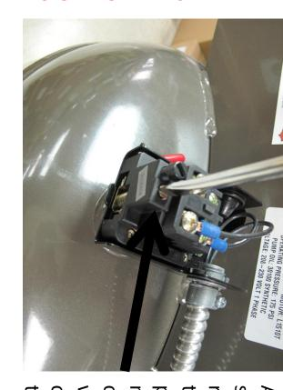
Adjust pressure set screw ¼ turn down to raise pressure or ¼ turn up to lower pressure (Do not adjust more than ¼ turn with out checking to see what the new operating pressure of the compressor is)
